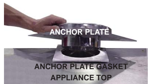
ANCHOR PLATE FOR A FACTORY BUILT CHIMNEY
