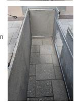
**6:** Square the connected panels and shim as needed. Connect 4 outside corners to panels by placing corners where side and end panels meet and pre-drilling holes into panels with a 1/4" masonry bit using existing holes in corners as a guide. Push bolts through corner and panel holes and use provided washer and nut to tighten bolt down. Do not over-tighten. Repeat until all corners are attached.
