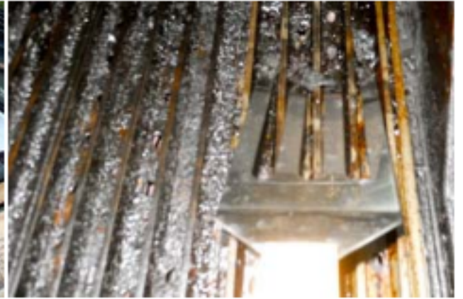
The GrateTool also shovels the debris.
