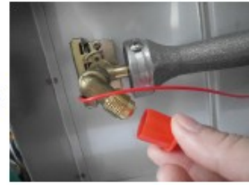
3.Remove the red sleeve
