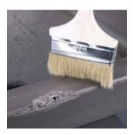
STEP 1: Clean surface of the damaged area by removing any loose material such as dirt, oil or grease and any loose of flaking cement pieces.
