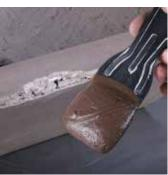
**STEP 2:** Thoroughly mix concrete mix as particles may have settled or separated during transport. (Mix should be lump free, putty consistency)
