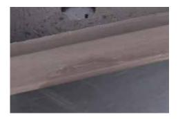
**STEP 5:** To remove excess concrete, with a damp sponge or rag, firmly wipe away the surrounding area, avoiding the newly filled area.
